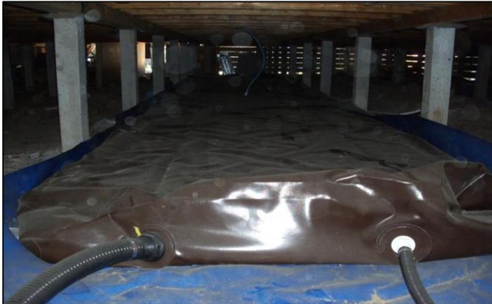
Fig 2. Showing the basic layout of a Rainwater Bladder.
